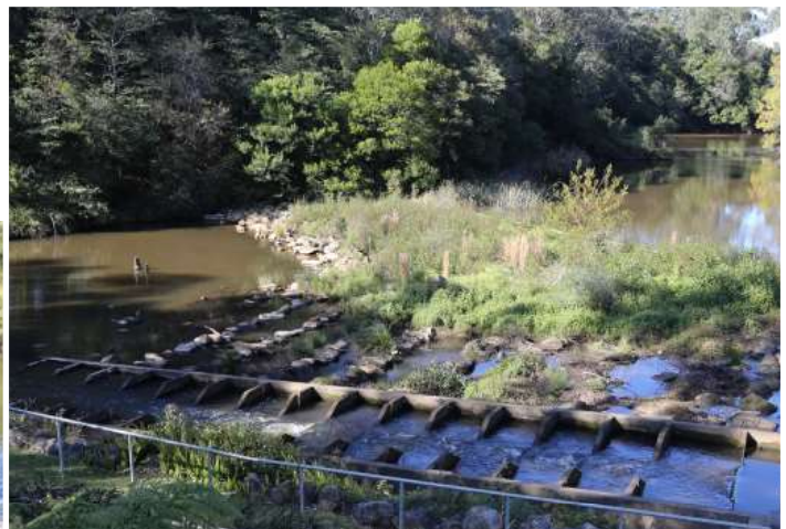
Wyong River Weir Fishway
