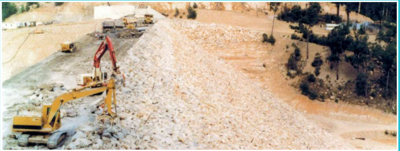
Construction of Mangrove Creek Dam wall
