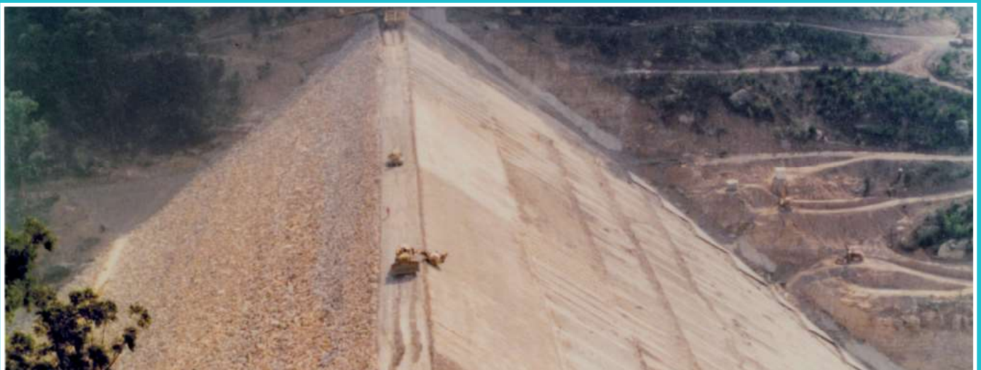
Mangrove Creek Dam wall prior to concrete
