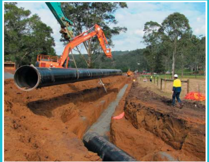
Mardi-Mangrove Link pipelaying
