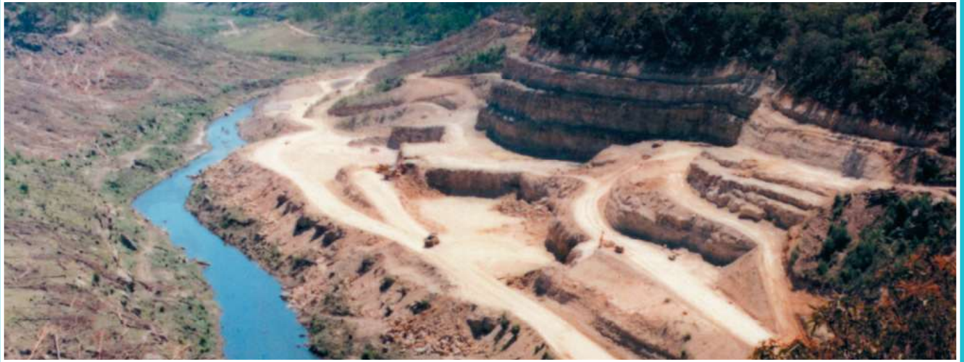
Mangrove Creek Dam construction quarry
