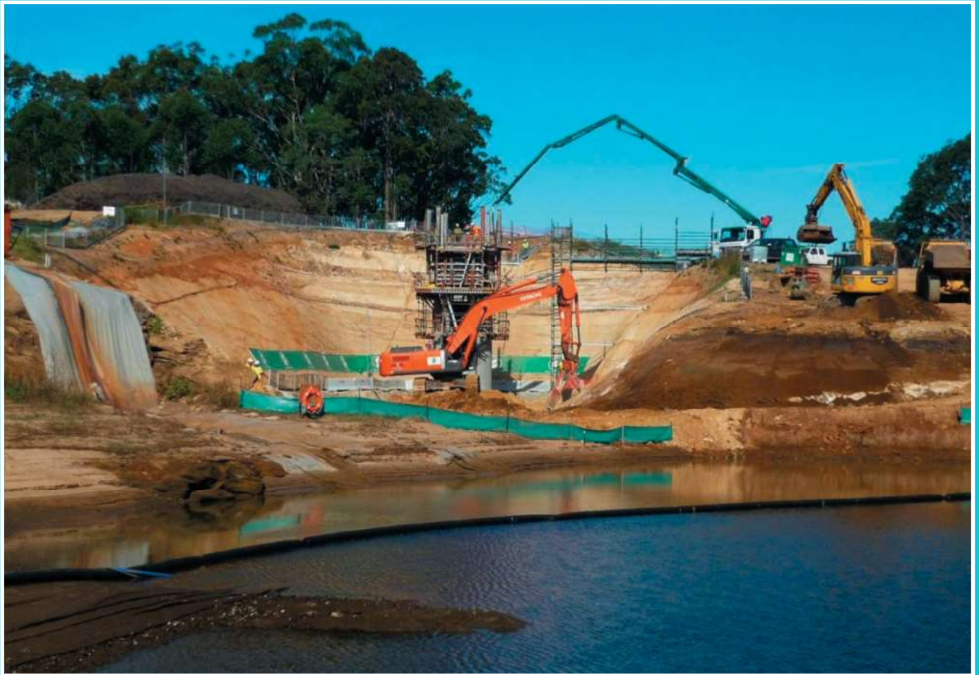
Construction of Mardi Dam intake tower
